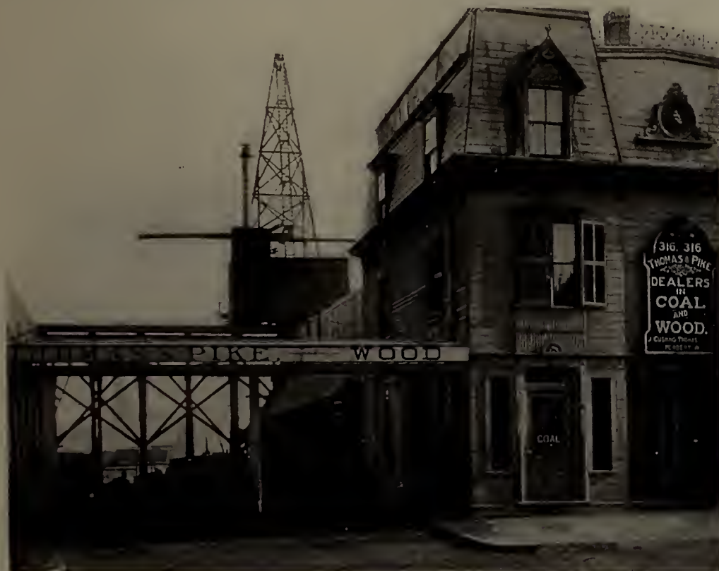
COAL YARD, OFFICE, AND ELEVATOR OF THOMAS & PIKE, 316 Albany Street. (J. Cushing Thomas, Herbert W. Pike.)
